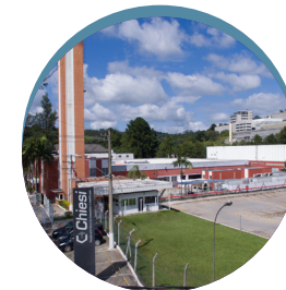
Santana de Parnaíba ISO 14001, ISO 45001 ISO 50001 (work in progress)
